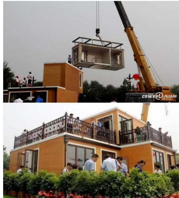
Fig. 7: Process of construction of the villa
